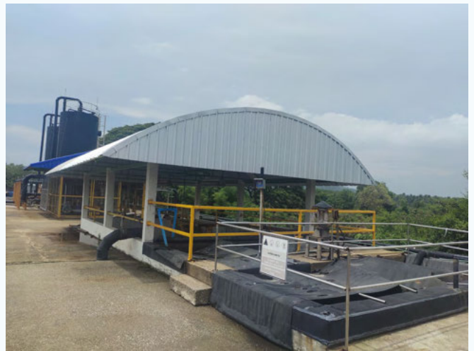
Changing the roof structure in the biogas pit area to prevent odor leaks and hazards associated with work activities in that area, thus extending the lifespan of machinery.
