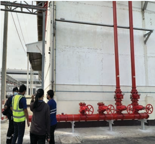
Implementing an automated fog water spray system in the warehouse to prevent and control initial stages of fire incidents.
