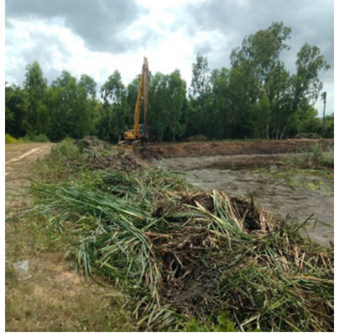
Dredging a Public Well in Nong Chok Sub-District, Nakhon Ratchasima Province
