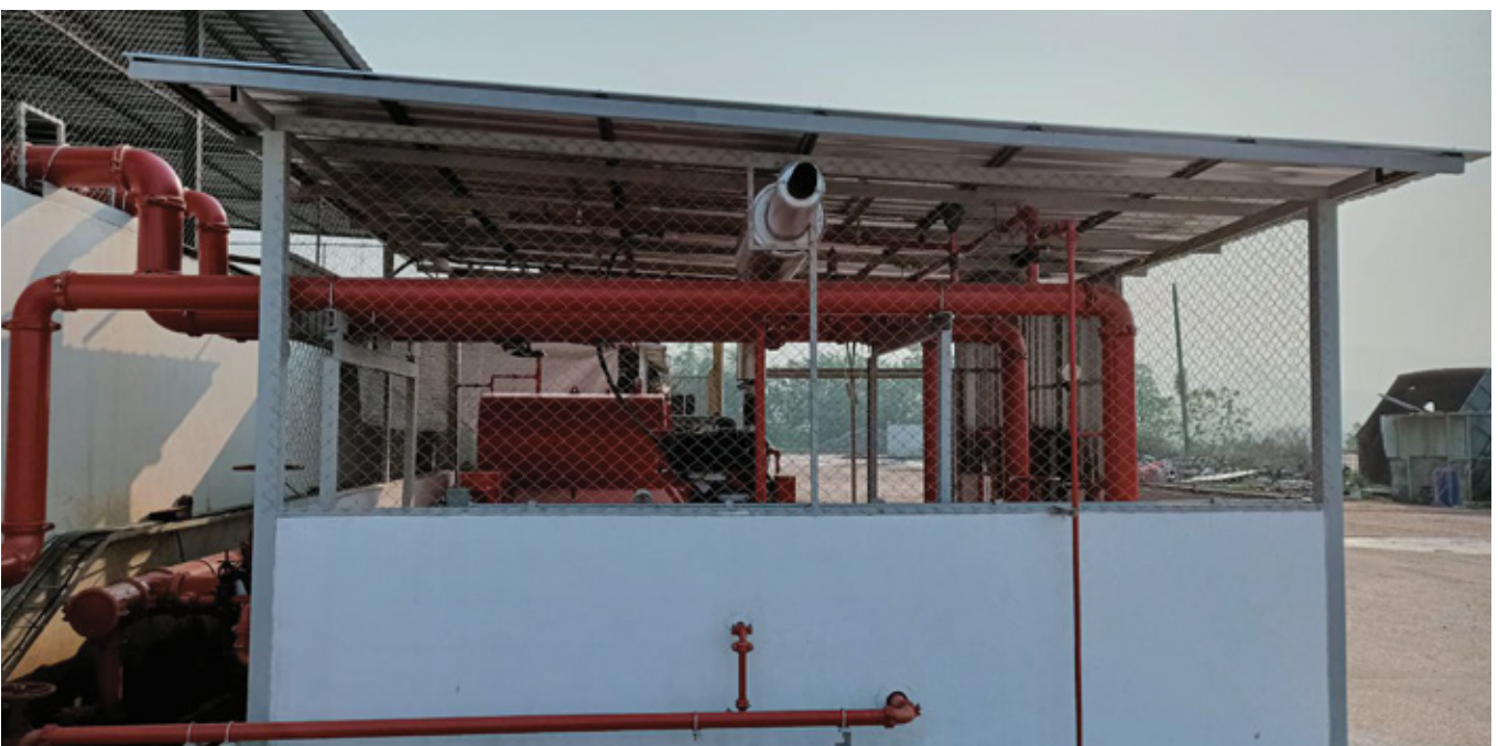
Installing Fire Pumpsto Prepare for Any Unexpected Emergency Situations
